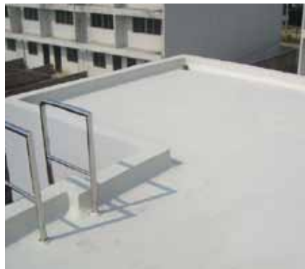
Finished roof waterproofing
