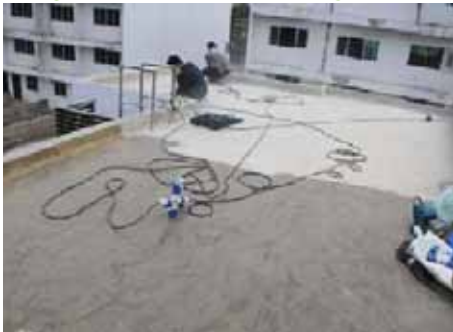
Preparation of the substrate
