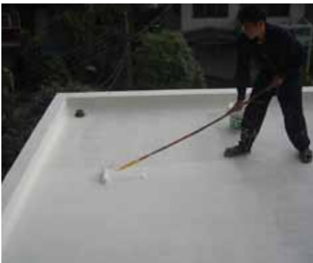
Application of the second layer. The KÖSTER Glass Fibre Mesh is embedded between the two layers.
