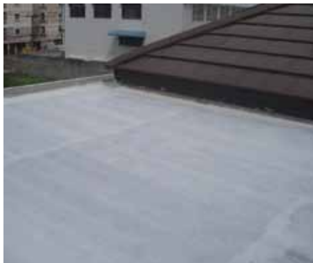
Application of the first layer
