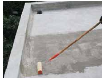
Priming with KÖSTER Polysil® TG 500
