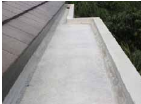
Installation of a concave fillet
